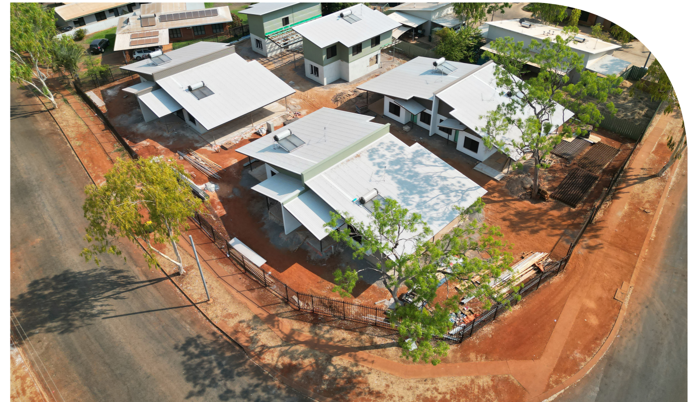
Image: Venture's new development in Katherine East will provide 8 new affordable homes.
